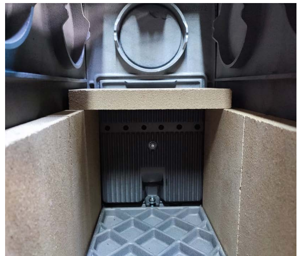
3. Put the top plates on top of the side plates.
